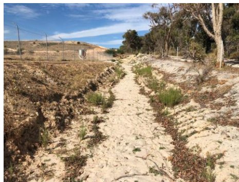
Image of drain lower than fire track in vicinity of evaporation ponds
