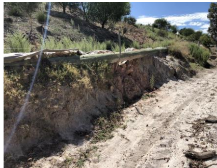
Image of failed drain flowing into adjacent fire track
